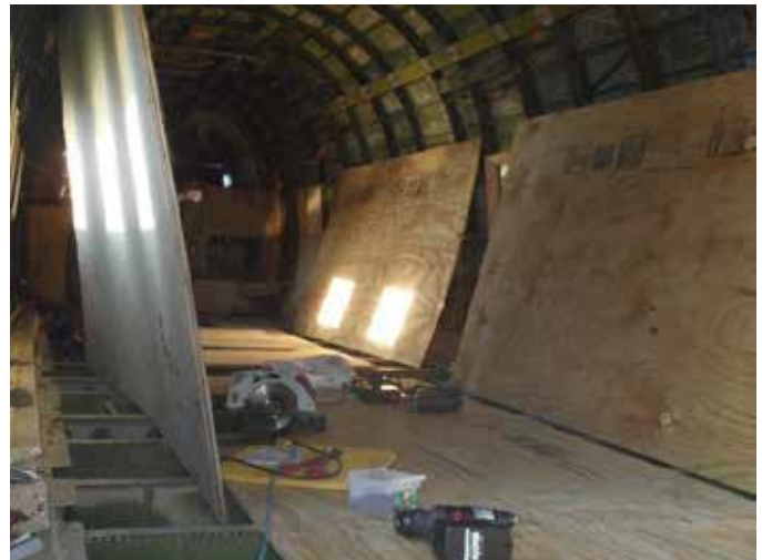
Interior stripped of all the rotted insulation, pressure washed, and being fitted with plywood.
